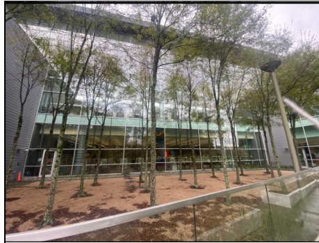
The exterior windows at the Main Goodwood East Baton Rouge Library that is the planned site for a window collision prevention solution.
